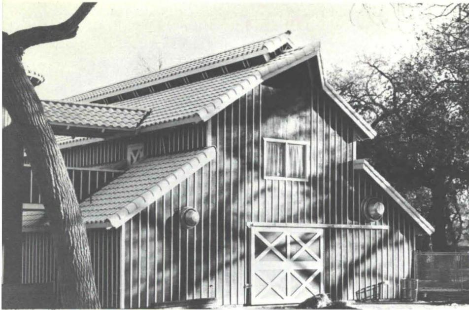
The new Childrens Barn.
